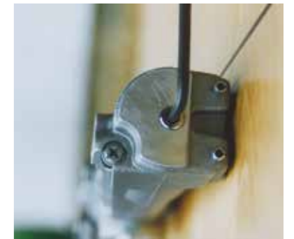
Briton 2003V power adjustment
