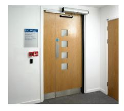
Touchless sensors are used to activate devices fitted to the main access doors to a surgery for example, allowing doctors and nurses to enter and exit the sterile area without touching any door handles or activation switches.
