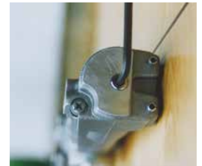
Briton 2003V power adjustment
